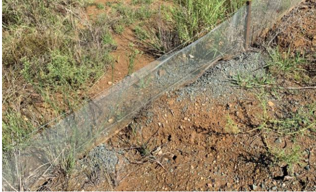
Figure 3: Soil eroded underneath exclusion fencing
