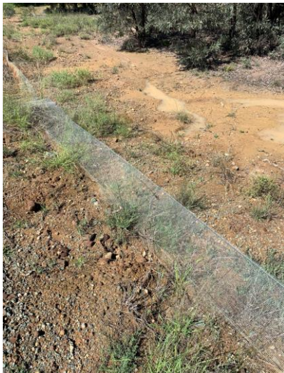
Figure 4: Damaged exclusion fencing
