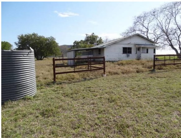
Figure 20: Site B15, Dovedale homestead in 2012 (Converge 2012).
