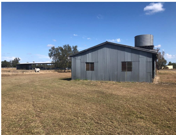
Figure 22: Sheds at the Broadmeadows homestead complex (AARC 2023).
