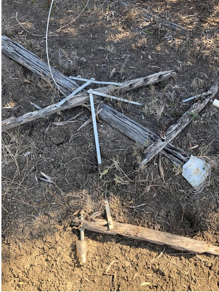
Figure 44: Example of cross bar with remnant insulators (AARC 2023).
