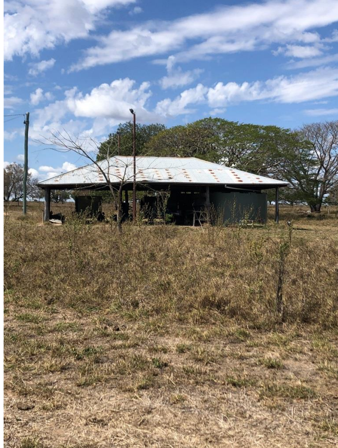
Figure 57: Shed to west of Dovedale homestead (AARC 2023).
