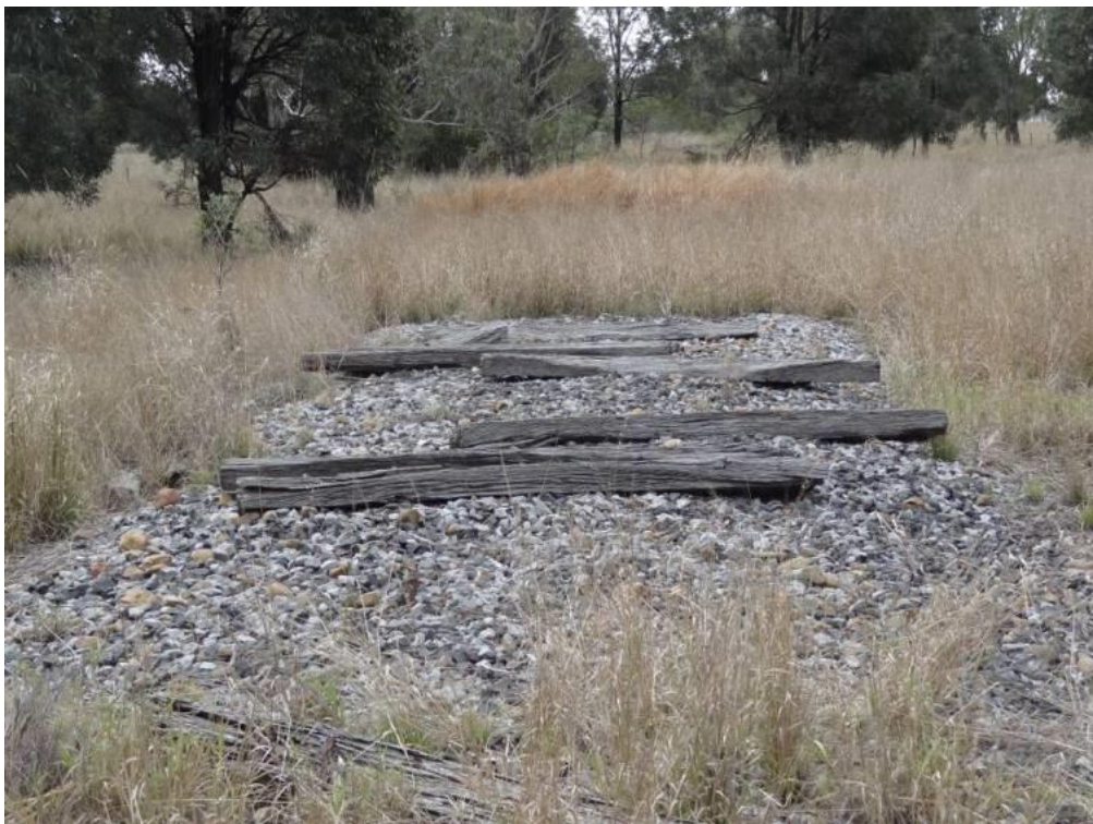
Figure 33: Example of remnant sleepers on embankment. View to the south (Converge 2012)
