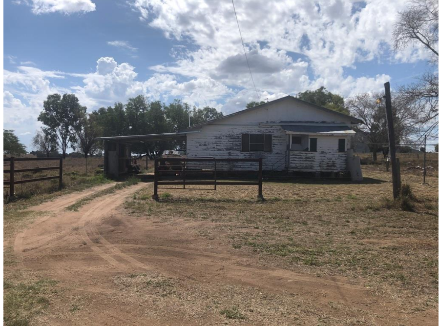
Figure 55: Dovedale homestead (AARC 2023).
